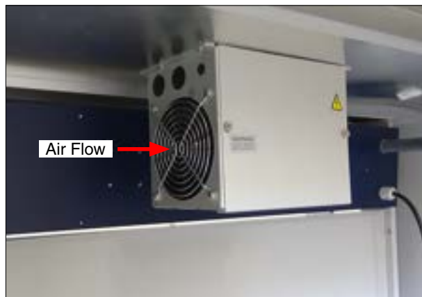
Figure 3.2h: Air heater fan housing under water pan.
